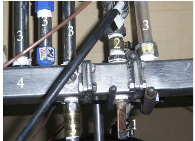
Fig. 6. Experimental assembling: 1 Cavity opposite the nozzle; 2 Input to the nozzle; 3 Additional cavities; 4 Air channel.
